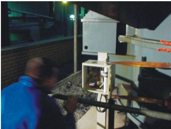
Fig. 3. Hall effect probe (white box) on transformer Earth line (copper) at Hunterston power station. Engineer (lower left) included for scale.
